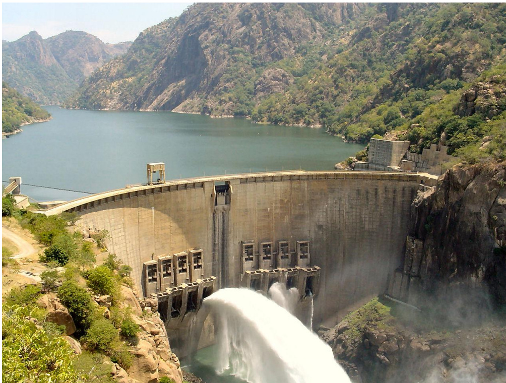
Figure 3- The Cahora Bassa Dam on the Zambezi River, Mozambique, with an installed capacity of approximately 2,075 MW the largest hydroelectric facility in the country and one of the largest in Africa
