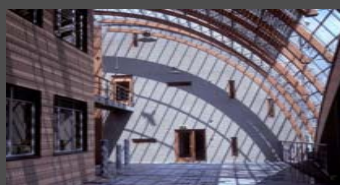
ECN Building 42.1, Peten, The Netherlands, 2001
