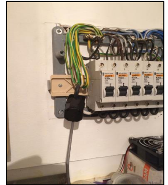
Figure 4 - Non-invasive current sensor
